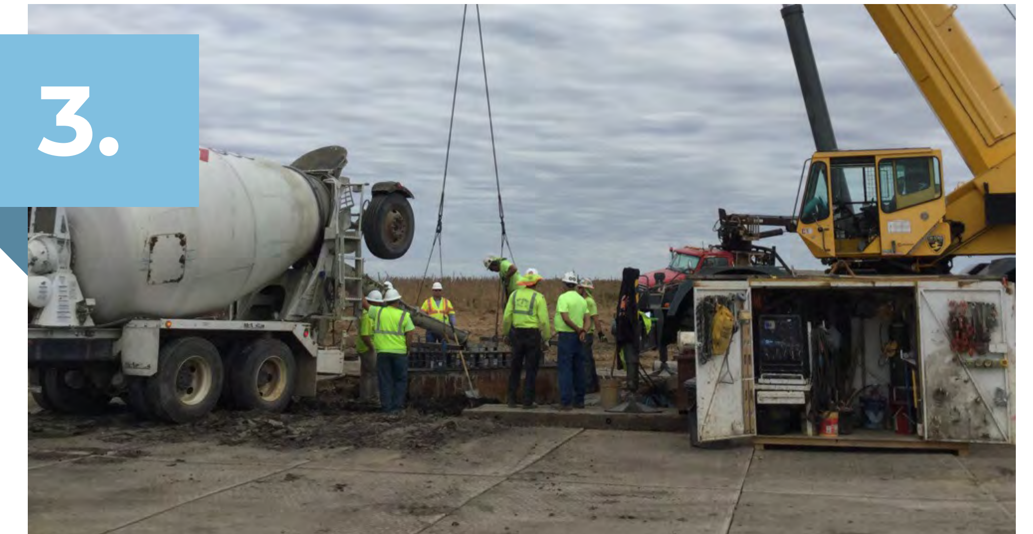
Foundation Drilling & Pouring
