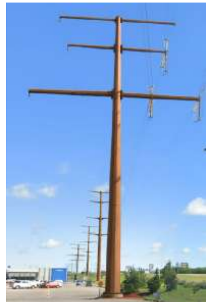
Double-Circuit Crossing Dead-End
