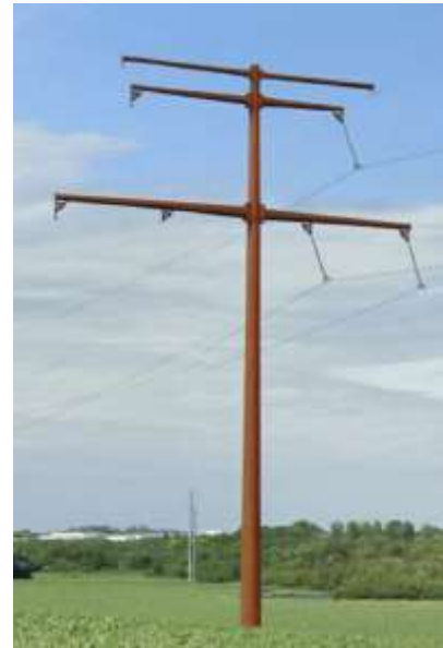
Double-Circuit Crossing Tangent
