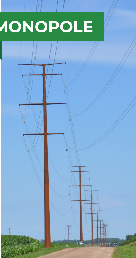
Image shown is an example of a similar double-circuit structure.
