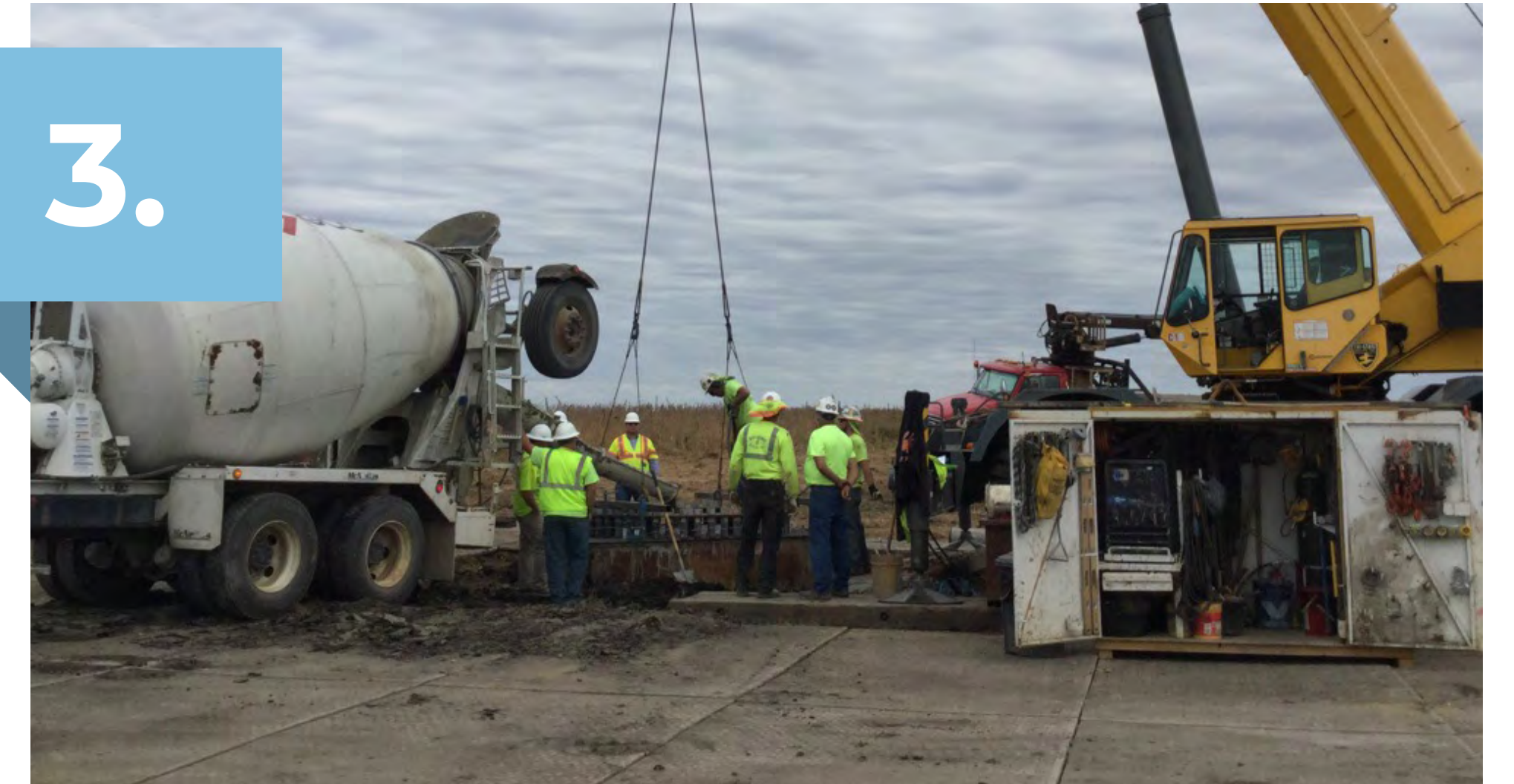
Foundation Drilling & Pouring
