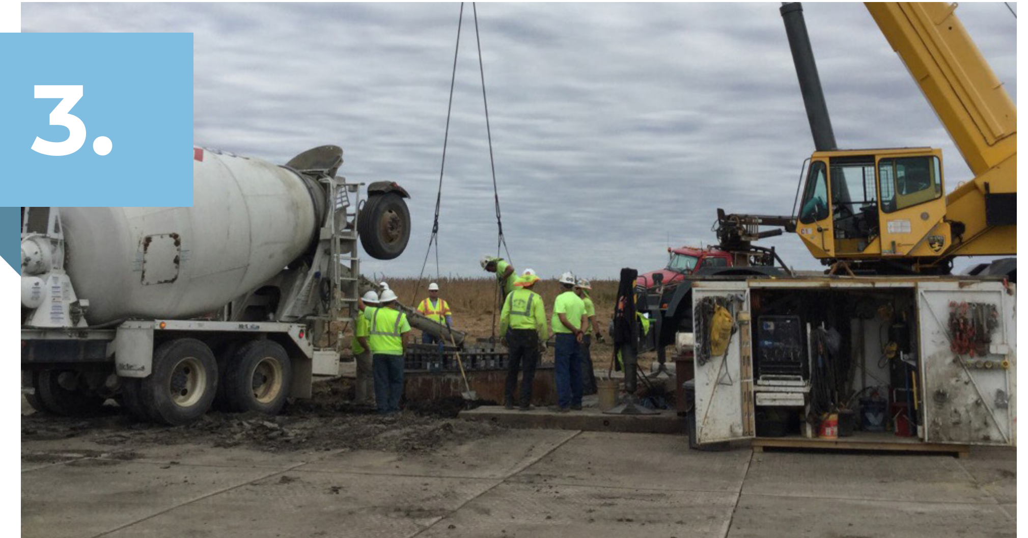
Foundation Drilling & Pouring
